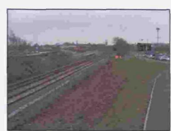
Proposed Location for Platforms & Station Building View Towards Coventry North Jn. (Feb. 2010)
